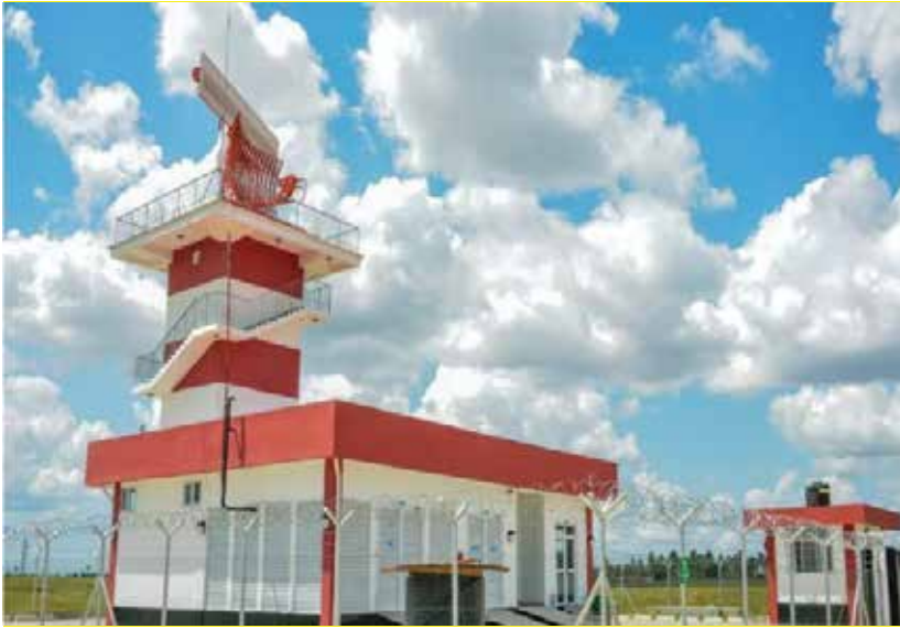
Figure 3: Dar es Salaam RADAR site
